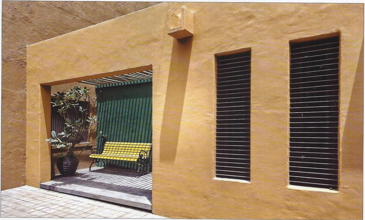
Bamboo Pergola outside Image Processing Unit & Studio
